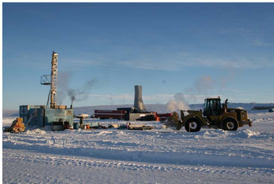
Figure 4: Core and large diameter rigs at site Q1/06
